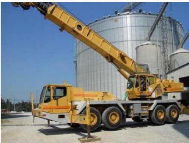
Figure 3. All-terrain, mobile, 50 ton crane.
